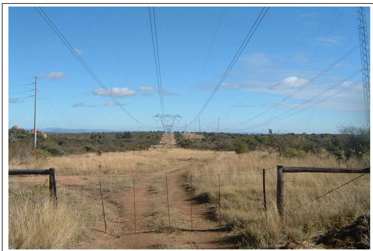
Figure 10- Option 04 for the proposed Mokopane Substation on the farm Noord Braband 774LR (above).
